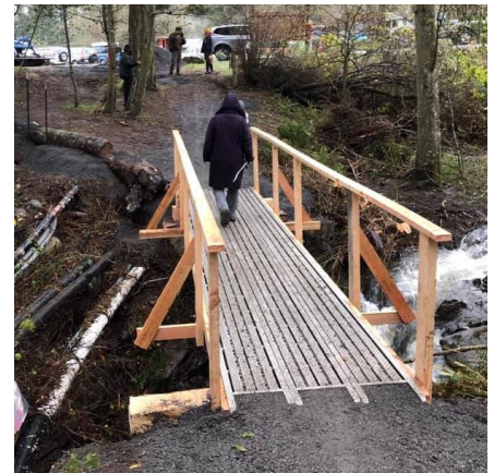
Foot bridge built by Orcas Island residents
